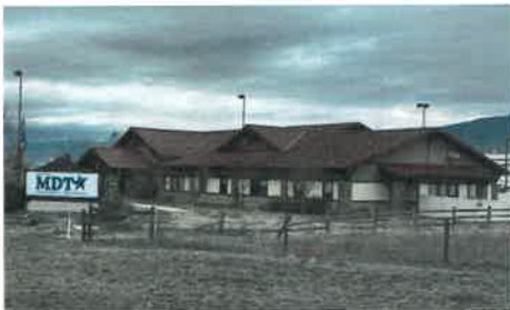
New Missoula District Headquarters building.
